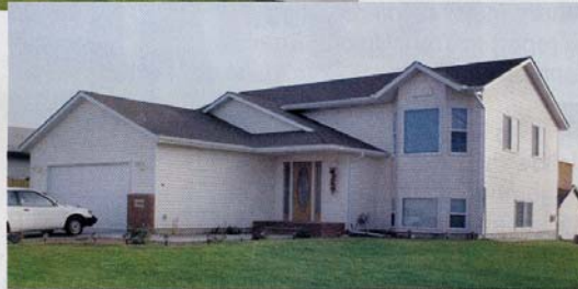
Pulis New Construction
