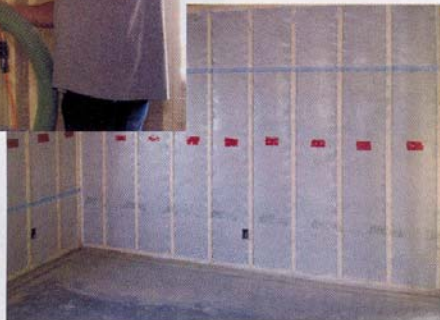
Pulis Staff Member applying the Par PAC Insulation System
