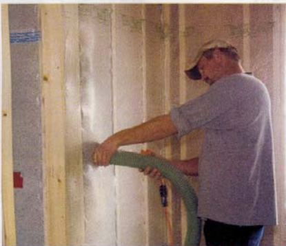
Pulis Staff Member applying the Par PAC Insulation System
